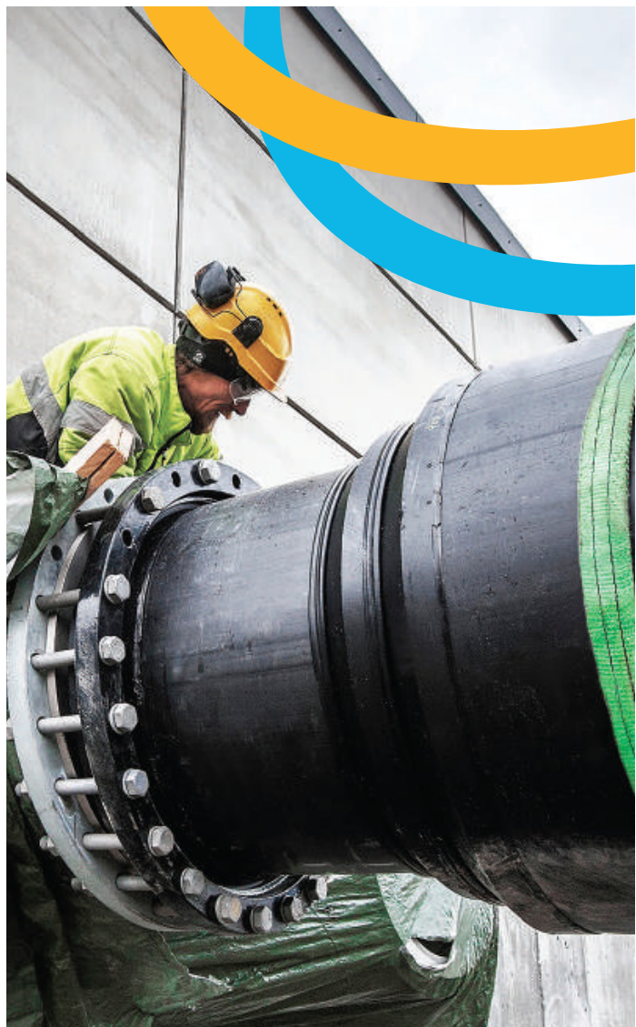
Figure 1: Typical flanged joint
