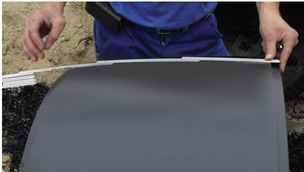
Figure 30: Measuring the coupler length
