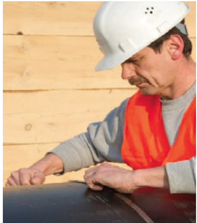
Figure 27: Checking the pipe diameter
