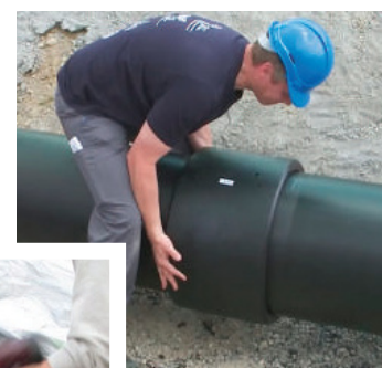
Figure 32: Sliding over of the coupler
