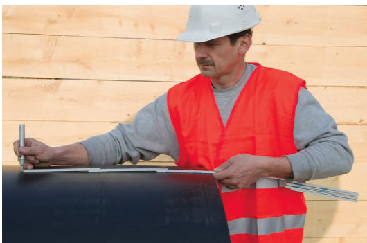
Figure 25: Marking the length for peeling
