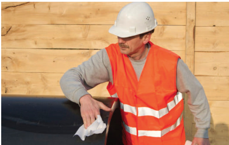
Figure 18: Pre-cleaning the pipe
