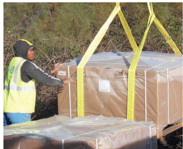
Figure 10: Transport of EF couplers d1200, packed on individual pallets in horizontal position
