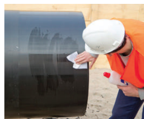
Figure 28: Cleaning of the fusion zone
