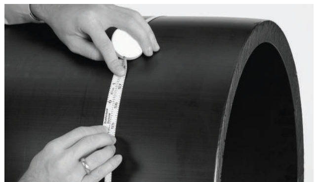
Figure 17: Checking the outer diameter of the pipe
