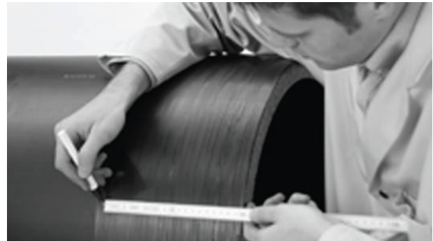
Figure 31: Marking the insertion depth
