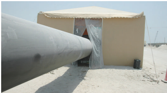
Figure 5: Protect the fusion area with a tent
