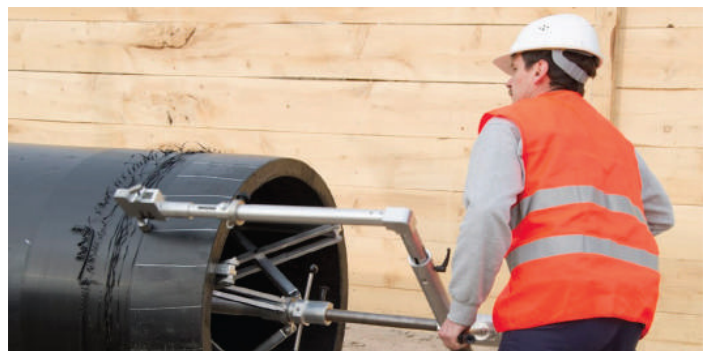
Figure 26: Peeling the pipe end
