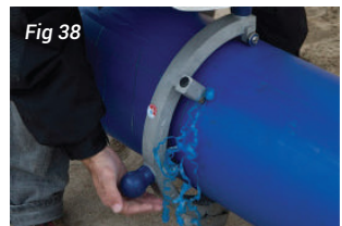
Figure 38: Rotary scraping tool
