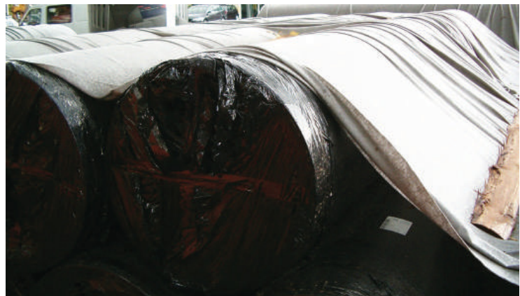
Figure 7: Protection of pipe against direct sunlight
