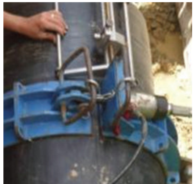
Figure 24: Hydraulic Re-Rounding
