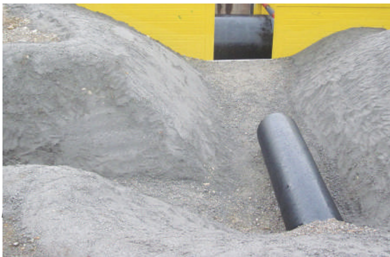
Figure 2: Pipe end excavated in a suitable length
