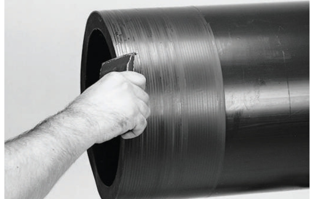
Figure 15: Deburr the pipe edge
