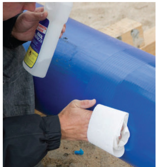
Figure 39: Cleaning of the scraped area
