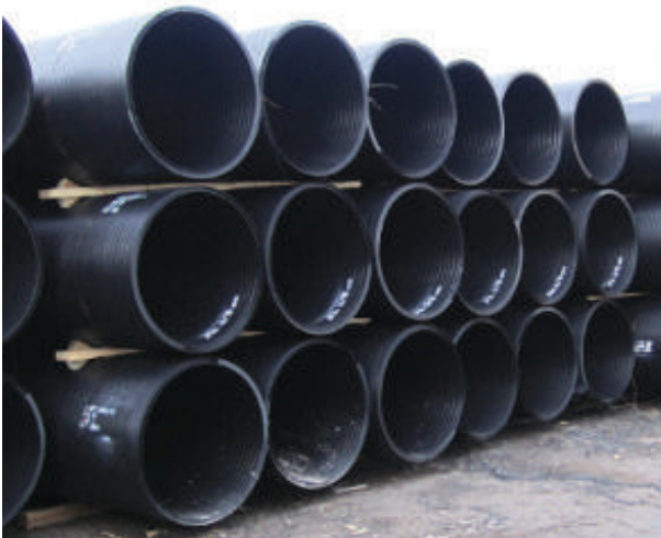
Figure 9: Example of good on-site PE Pipe Packing and Storage
