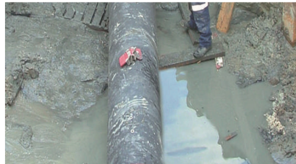
Figure 6: Ground water has to be pumped out from the working pit
