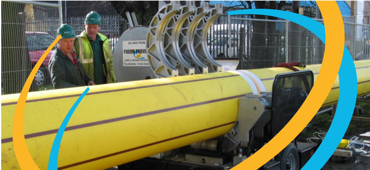
A fully automatic butt fusion welding machine for 630mm diameter polyethylene pipe systems Image courtesy of Radius Systems Ltd
