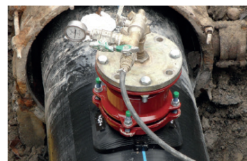
Fig. 19 Wide range restraint coupling used for a pressure test on a branch connection.
