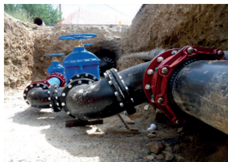
Fig. 14 Flange connections in the field
