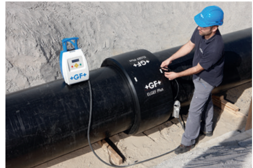
Fig. 11. Electro fusion machine welding a big dimension coupler
