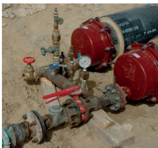
Fig. 20 Wide range restraint end caps
