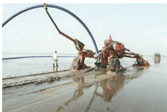
@ Walter Foeckersperger GMBH Picture: Flexible PE100-RC pipe installed directly into the ground without open trench
