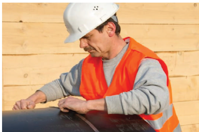
Figure 27: Checking the pipe diameter
