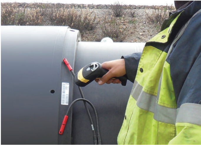
Figure 34: Scanning the fusion bar code
