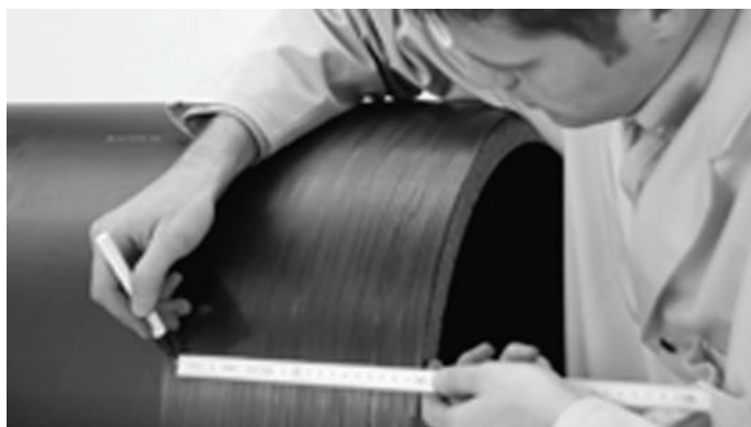
Figure 31: Marking the insertion depth
