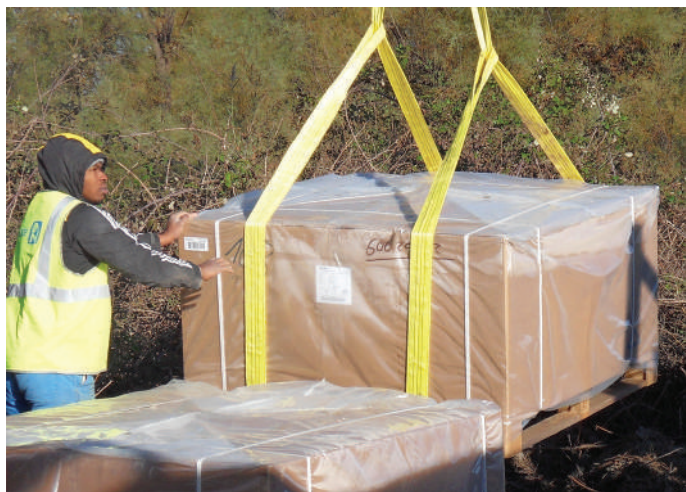
Figure 10: Transport of EF couplers d1200, packed on individual pallets in horizontal position
