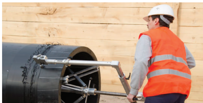
Figure 26: Peeling the pipe end
