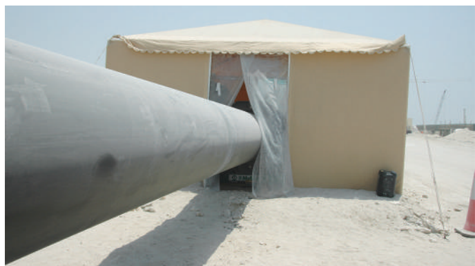
Figure 5: Protect the fusion area with a tent
