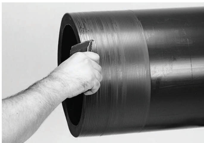
Figure 15: Deburr the pipe edge
