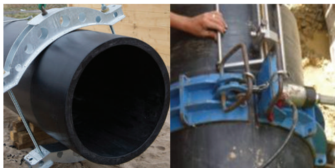
Figure 23: Mechanical Re-Rounding / Figure 24: Hydraulic Re-Rounding
