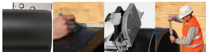
Fig. 19 Toe-in of pipe ends, Fig. 20 Marking the cutting position, Fig. 21 Cutting the pipe end / Fig. 22 Deburr the pipe end
