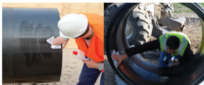
Figure 28: Cleaning of the fusion zone / Figure 29: Cleaning of the EF coupler
