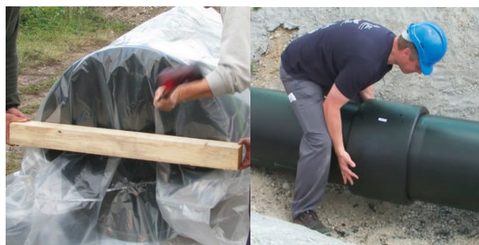
Figure 32: Sliding over of the coupler
