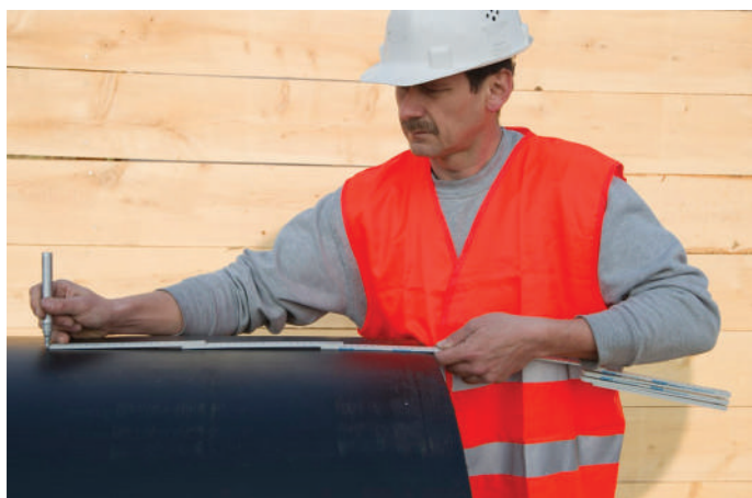
Figure 25: Marking the length for peeling
