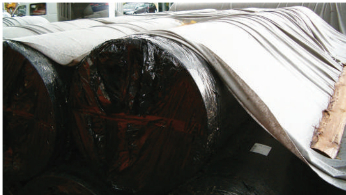
Figure 7: Protection of pipe against direct sunlight
