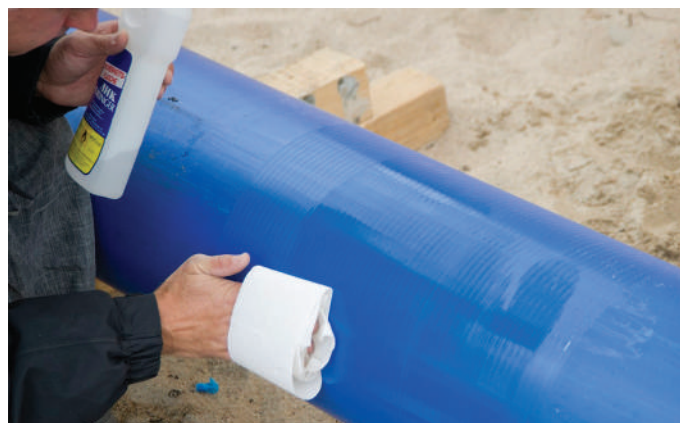
Figure 39: Cleaning of the scraped area
