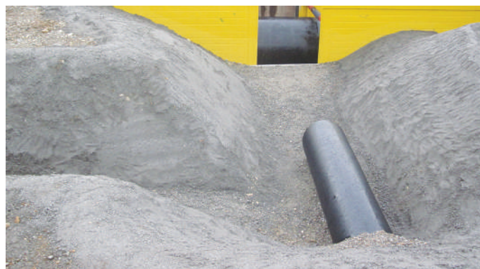
Figure 2: Pipe end excavated in a suitable length
