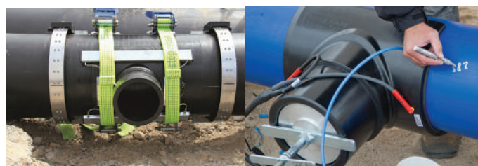
Figure 40: Mechanically clamped system
