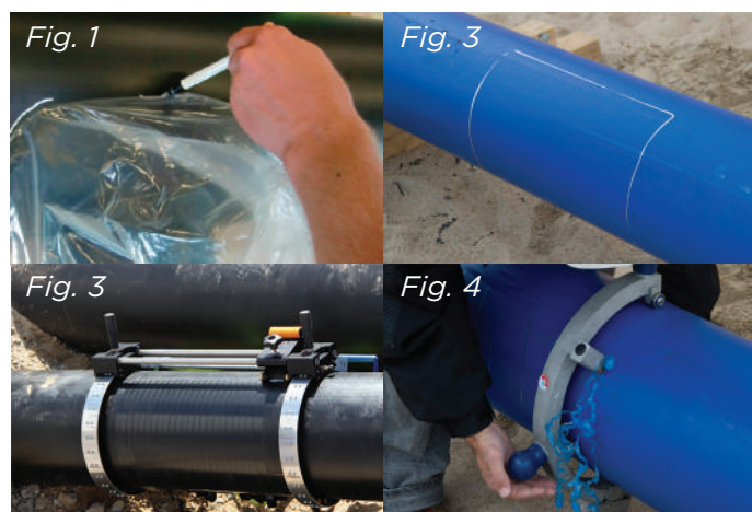
Figure 35 & 36: Marking the area for scraping
