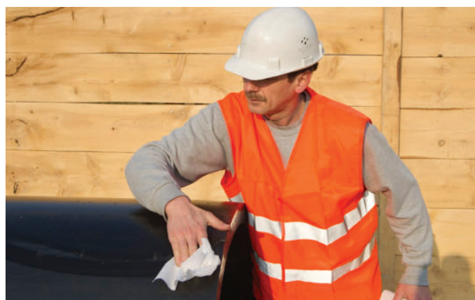
Figure 18: Pre-cleaning the pipe
